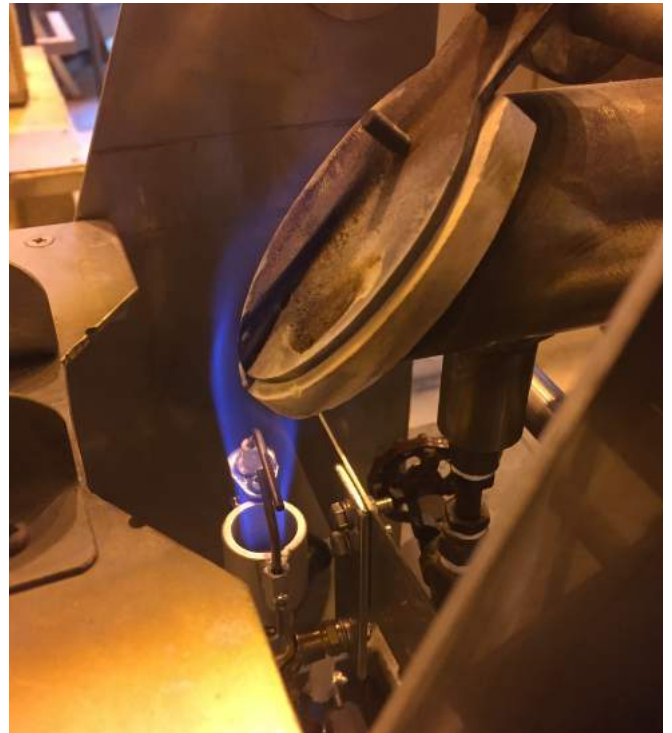
The AIPB mounted on a furnace and used to flare off Hydrogen.
